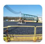
The hollow plastic balls that form a floating cover for ponds, tanks, lagoons, and other basins.
