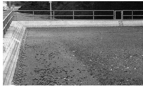
Seep tank on a compost plant covered with ALLPLAS balls PP, Ø 70 mm, black.
