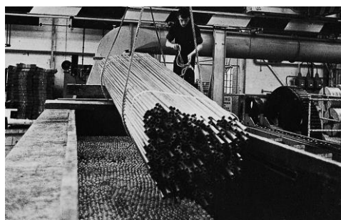
ALLPLAS balls covering a hot processing tank in an aluminium plant. The floating ball blanket ensures that surrounding machinery and equipment remain in perfect and fully operational condition.
